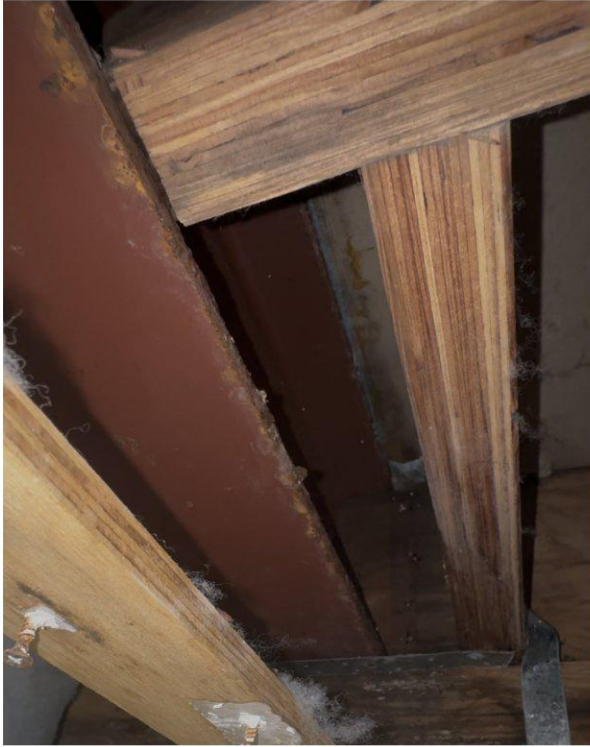
Photo 9 — Joists and framing in cavity around beam
